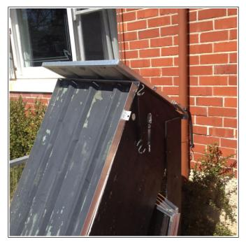
The roof top is lose, kept down with straps, but also adjustable down, so when very stormy can close it more or less fully so no water comes in, still leave a little gap.
